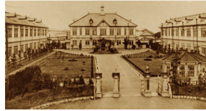
落成直後の奈良女子高等師範学校正面（大正2年） The front view of Nara Women's Higher Normal School soon after its completion (1913)
